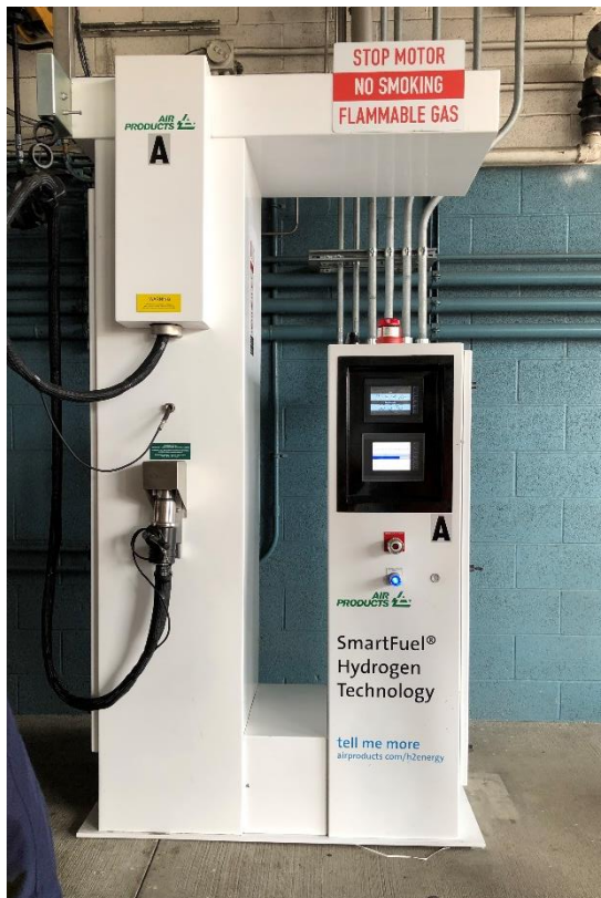
Figure 26: Hydrogen fueling dispenser at OCTA for heavy-duty transit buses
